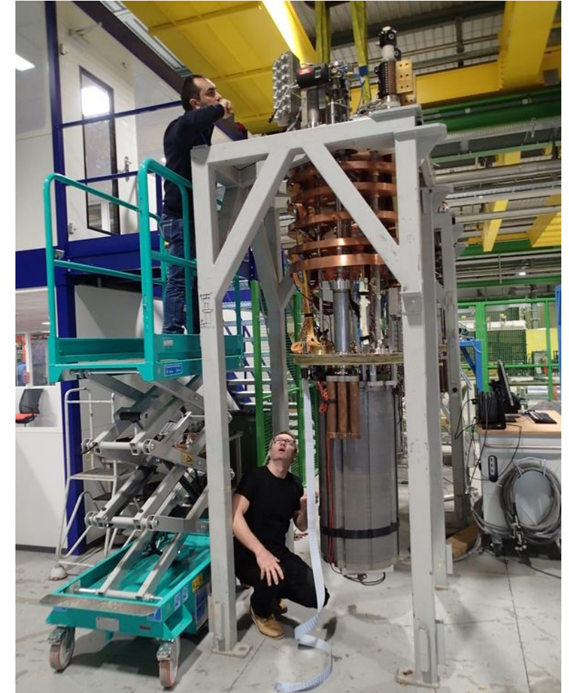
The test facility for superconducting structures and LHC magnets installed inside
