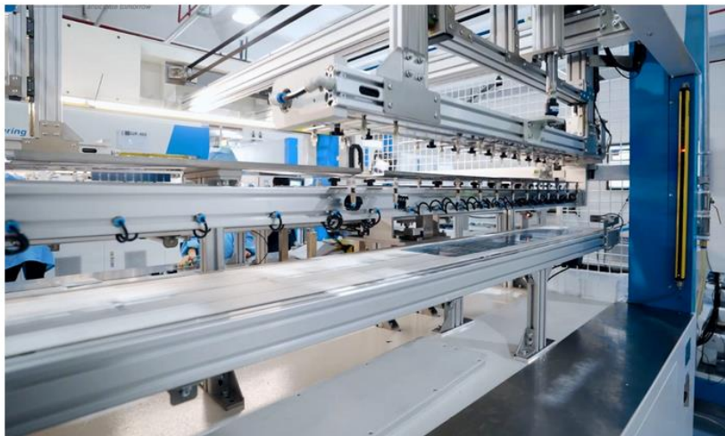
The new factory will also include an R&D centre and a test field for product control and improvement. Image: FuturaSun
