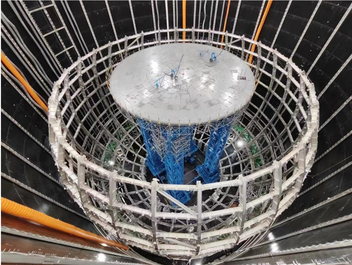
Installation platform finished (May 2022)
