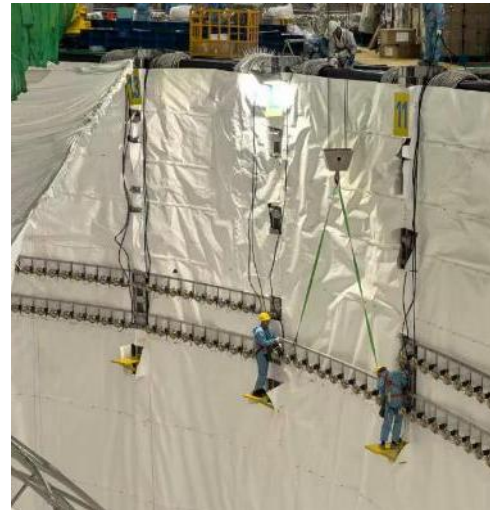
PMT and Underwater box installation
